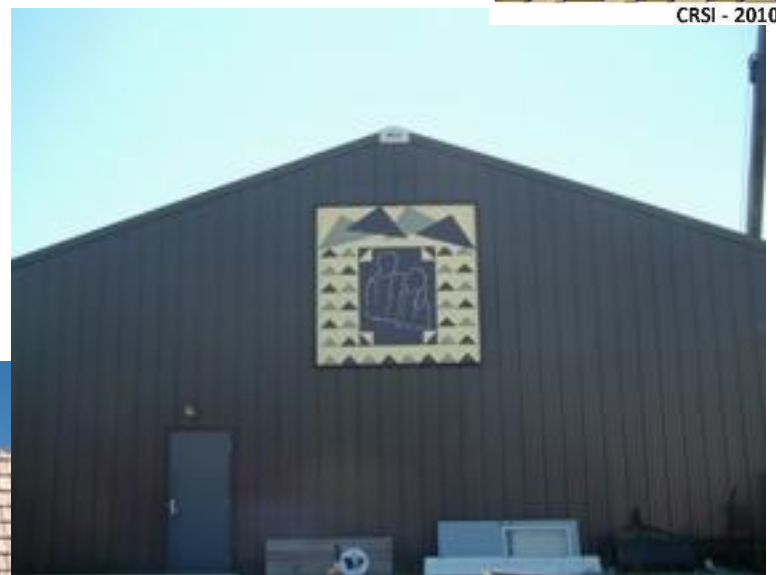
Corporate Office Maintenance Barn Rear Entrance U.S. HWY 36
