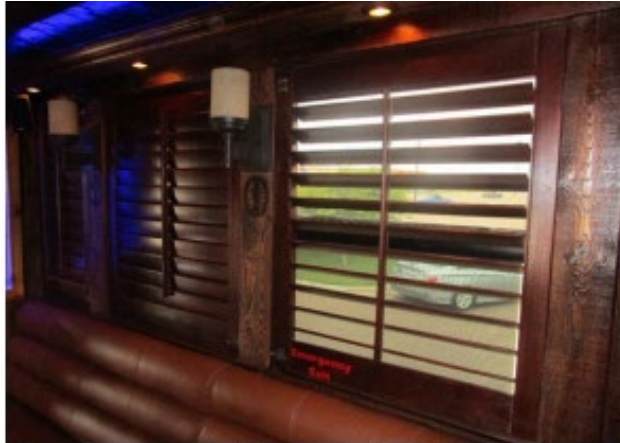
Exit obstructed by wooden plantation shutters.
